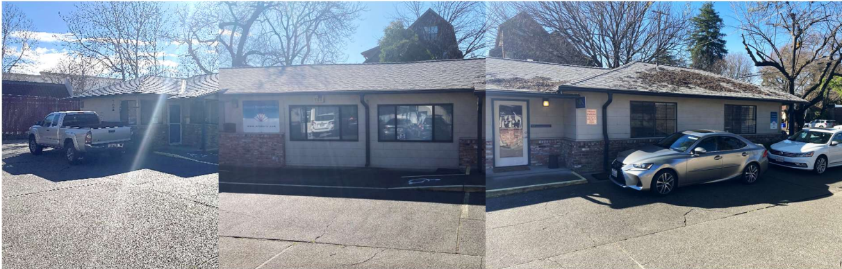
Secondary (north) façade, composite view facing south. Source: ESA, 2024.
